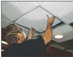
Remove Old Panels
